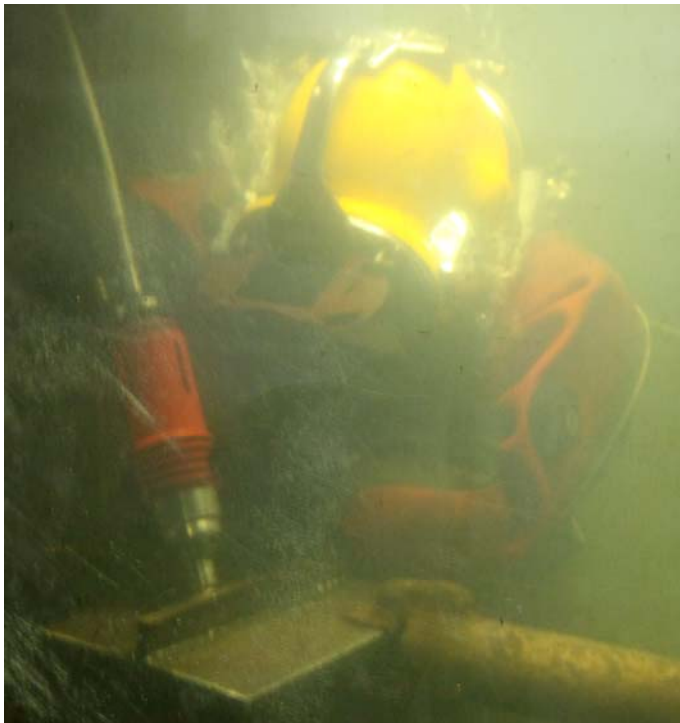
Fig.1b. The process of underwater ultrasonic peening by using of the specially designed tool
