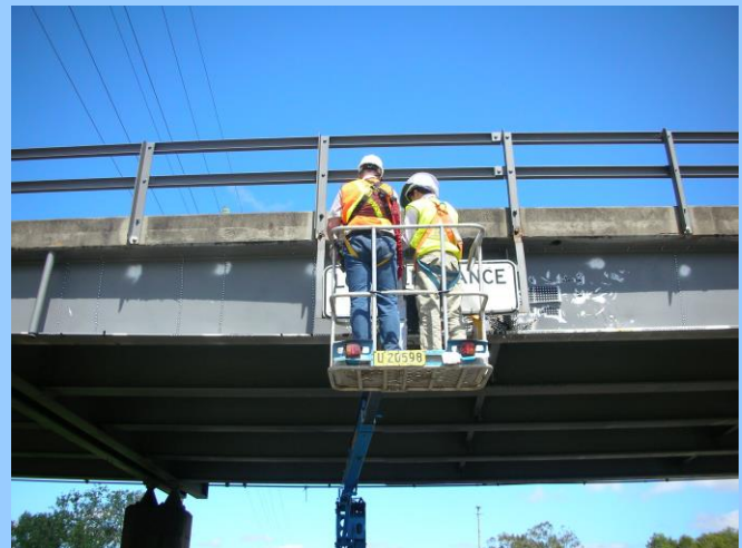
Use of the UltraMARS ® system in a field project for evaluation of distribution of residual stresses on a transportation bridge in Australia.
